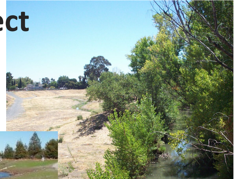
Reach 6 Channel Widening
